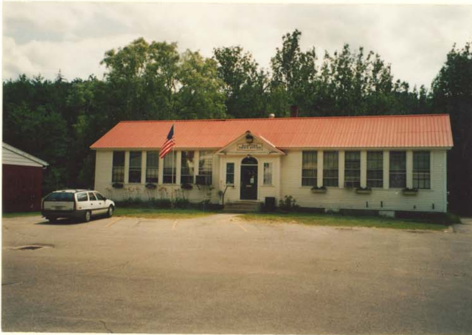
Campton Town Office Building
